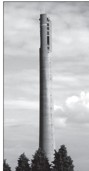
Figure 1. National Lift Tower
